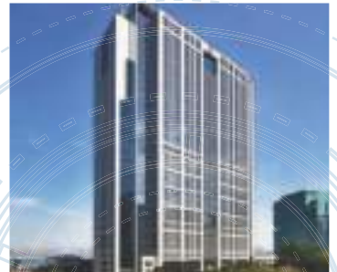
Customs Headquarters Building, Hong Kong
