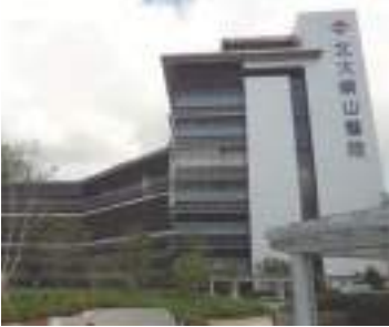
Lantau Hospital, Hong Kong
