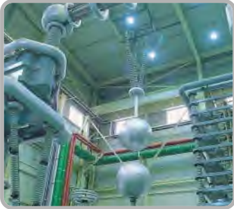
High Voltage Test / Impulse Test
